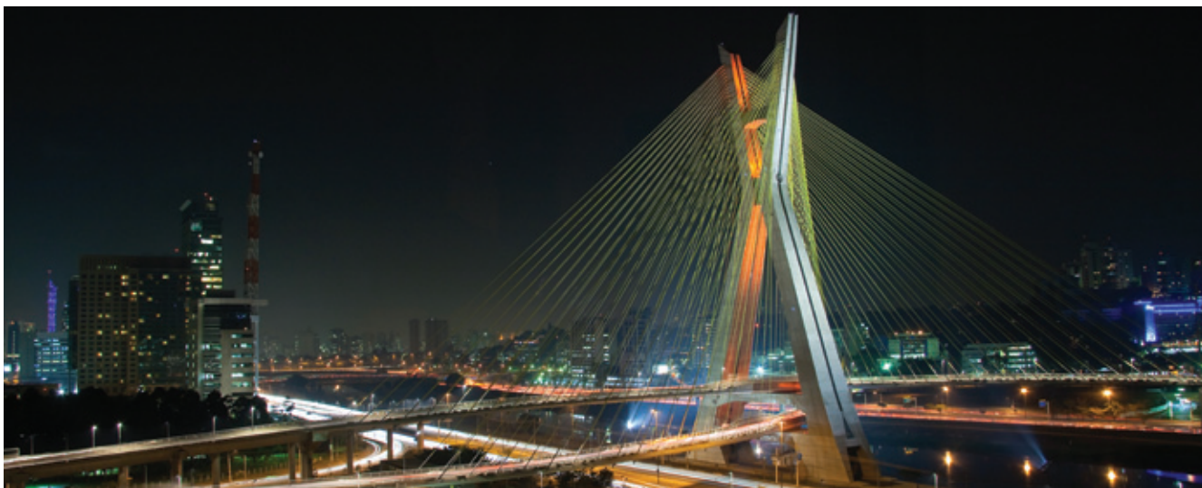
▲ Photo credit: www.bigstockphoto.com 'Octávio Frias de Oliveira Bridge', São Paulo, Brazil Photographer: Celso Diniz
