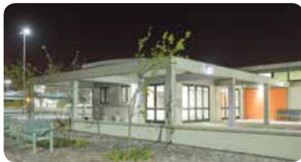
SERIES LED bulkheads were installed around the exterior of the buildings.
