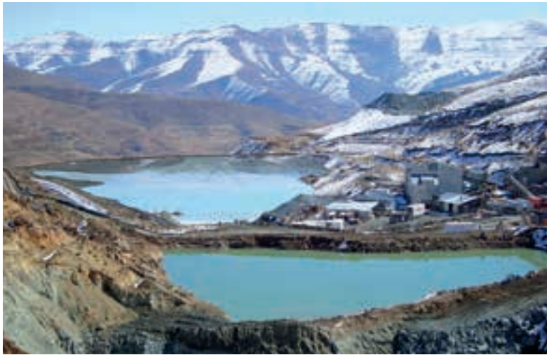
This is how the Liqobong site looked several years ago. The old plant seen here was dismantled and removed prior to the start of construction of the current project.
