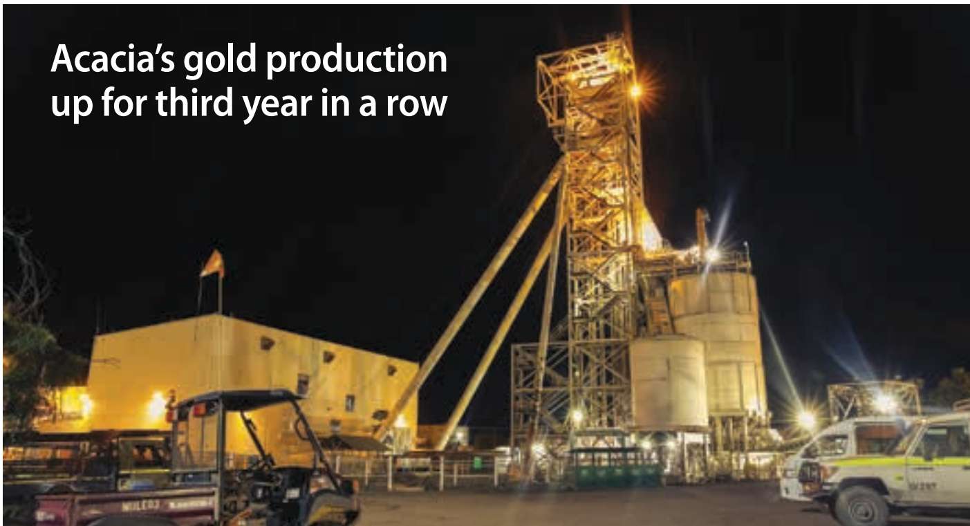
The Bulyanhulu gold mine. Acacia has fundamentally re-engineered the operation at Bulyanhulu over the past two years and delivered a 40% production increase in that time (photo: Acacia).
