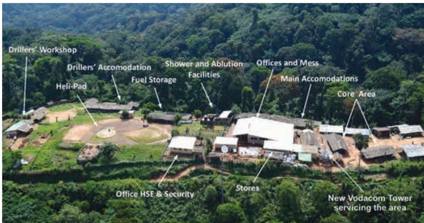
The camp serving the Bisie project in the DRC's North Kivu Province (photo: Alphamin).
