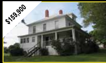
$159,900 MLS 61469 RURAL RETREAT 3BD/2BA updated farmhouse that is a must see. Lg rms including a kitchen, DR with french door opening to the LR and a library. Wrap around country porch to enjoy. New heat pumps, wiring and plumbing. Call today.
