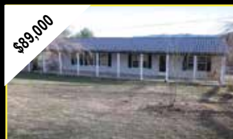
MLS# 58791 WYTHEVILLE 3BD/2BA home on over 1/2 ac. SS appliances, Master suite has 2 walk in closets, full BA w/ double sinks, garden tub, & shower. Concrete porch on front and one side.
