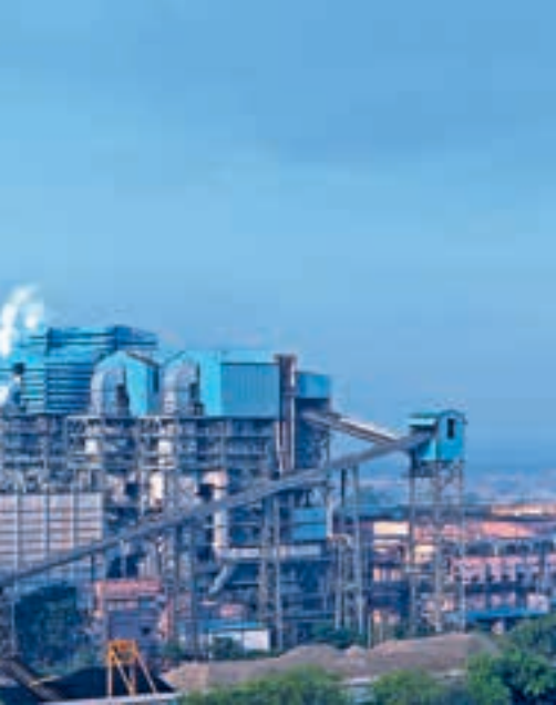
Above: The thyssenkrupp Industrial Solutions Service Centre in Chloorkop, originally equipped to manufacture and refurbish the largest Polysius-branded HPGRs, has CNC vertical and horizontal machining centres capable of handling 100 t components. Left: thyssenkrupp's coal-based circulating fluidised-bed combustion (CFBC) power stations operate at lower combustion temperatures and subcritical steam conditions. They can use much lower quality coal and discard coal, for example, which is normally regarded as unusable.
