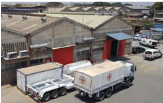
ABB is to provide a hybrid solar-diesel microgrid to power the Kenyan logistics hub of the International Committee of the Red Cross (ICRC).
