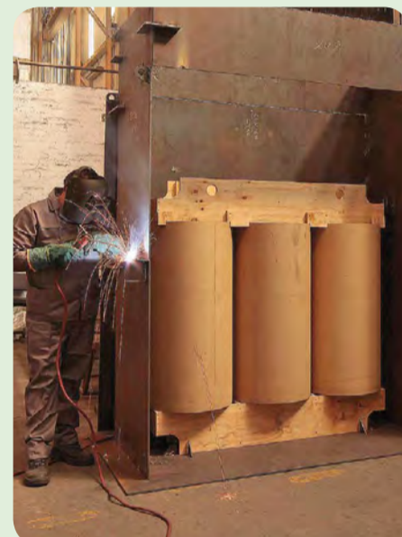
A welder works on a full-scale model that was made to facilitate achieving the optimum design for the new wind farm transformers.
