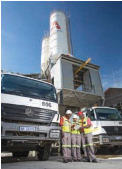
AfriSam operates a fleet of 50 ready mix trucks and two sophisticated boom pump vehicles in KZN.
