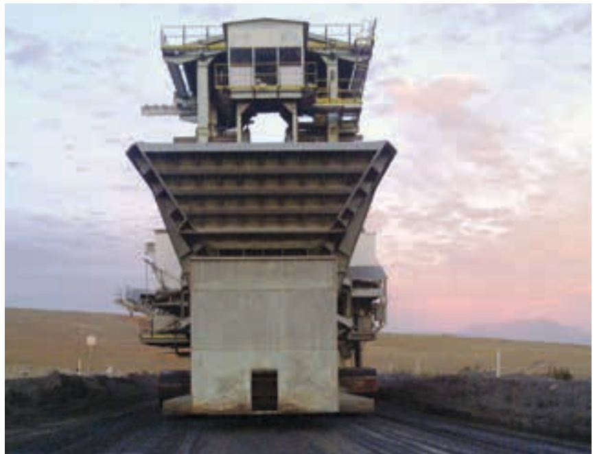
The primary crusher is a semi-mobile unit, which is moved to the service area every three to four years for maintenance purposes (courtesy PPC De Hoek).
