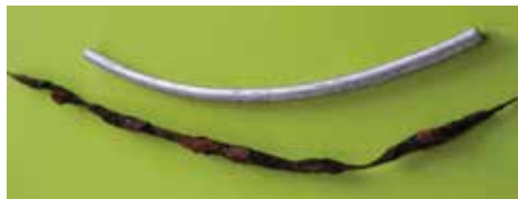
Figure 1: Corrosion of 10 mm solid galvanised conductor – after eight years.
