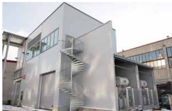
The utility-scale solar inverter laboratory, located in Helsinki, Finland.
