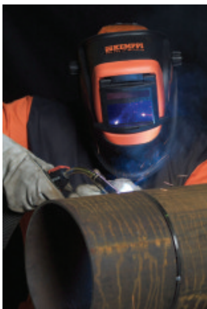
FastMig Synergic welding of pipe using Kemppi's FastROOT software
