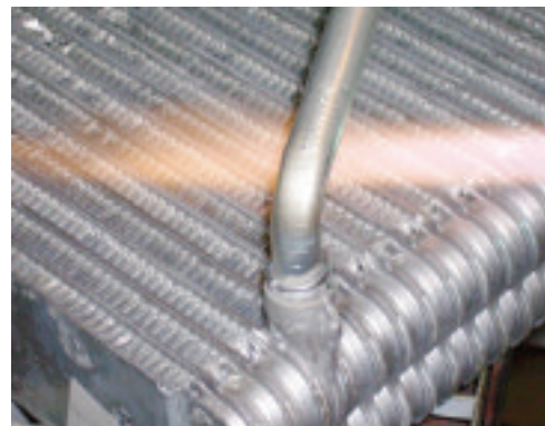
① Pipes brazed to radiator fittings using Total Brazing Mix™
