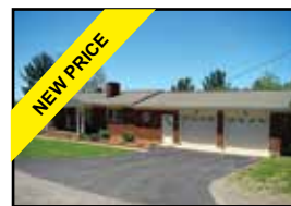
MLS 60119 - Hillsville - 4 BR, 2 BA, 2000 Sq. Ft., 16 acres, laminate wood floors, remodeled, new kitchen cabinets/appliances, new BA fixtures & tile, brick FP, large 2 car garage, separate carport, mountain views. $159,000
