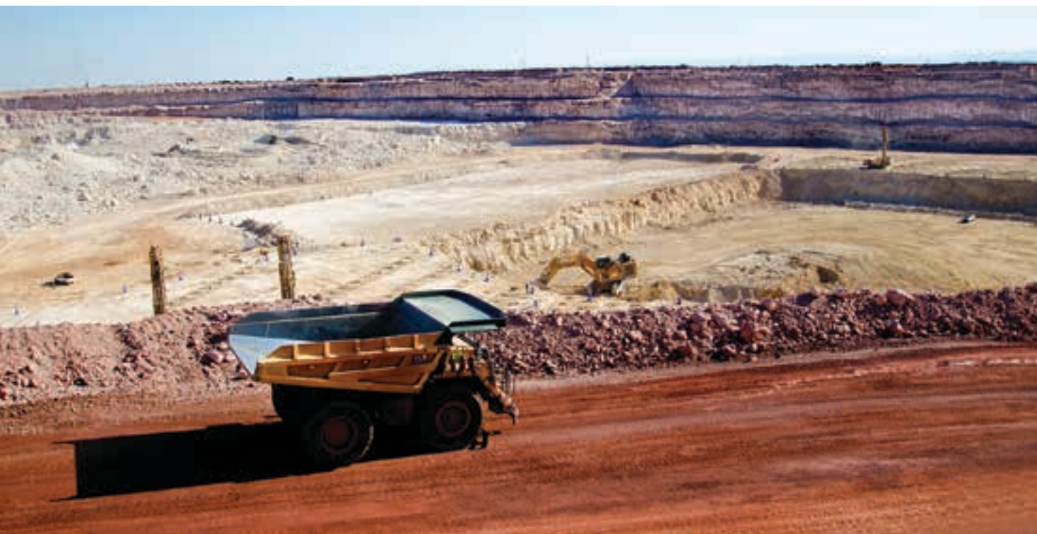
Cat 777F dump truck working at the Klipbankfontein pit, Kolomela iron ore mine in the Northern Cape.
