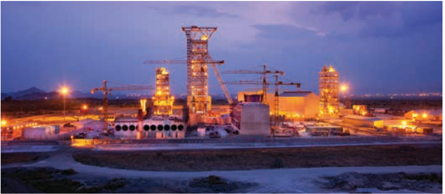
Impala Platinum says that the capital expenditure programme for No 17 Shaft (seen here) will be slowed to conserve cash, prioritising the completion of the main shaft-sinking programme.
