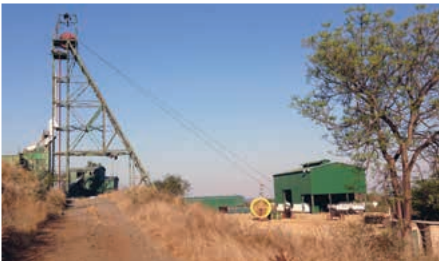
The Blanket gold mine near Gwanda in Zimbabwe showing the No 4 Shaft headgear. The mine is to sink a new 6-m diameter Central Shaft from surface to 1 080 m (photo: Caledonia).
