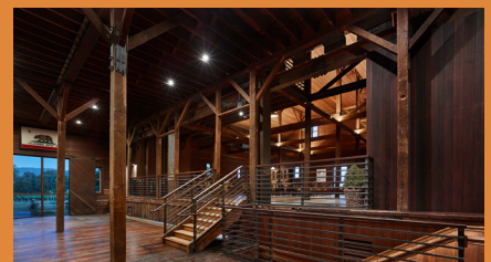
May 2017 - After a full restoration, including a modern seismic retrofit, our historic winery is ready to stand sentinel over Napa Valley once again.
