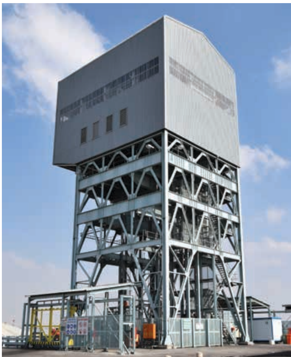
The main shaft headgear at Impumelelo.
