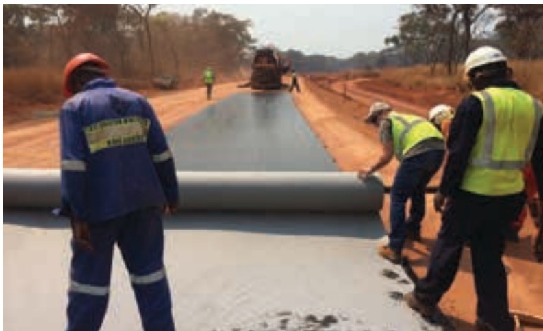
Fibertex AM-2 paving fabric has been used in a recent road surfacing project in Zambia.
