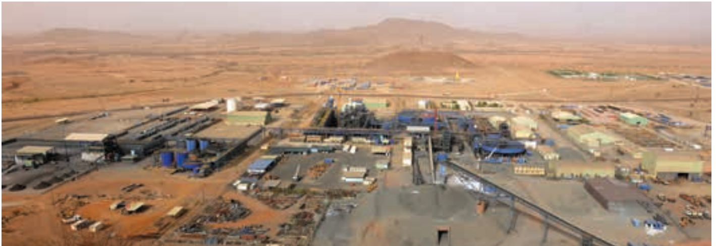
View of the Bisha site. Starting from the left of the photo and moving towards the centre, the concentrate storage, filtration, thickening and flotation sections of the zinc flotation plant expansion can be seen (photo: Nevsun).
