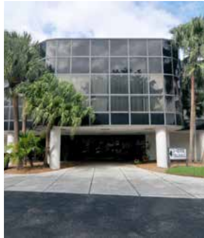
AT&T REGIONAL Fort Lauderdale, Florida 79,412 SF $4,900,000 Bridge Loan
