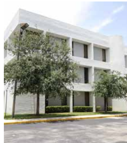
WELLS FARGO BANK BUILDING Delray Beach, Florida 15,890 SF $1,775,000 Permanent Loan
