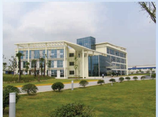
The facilities of Changshu Walsin, a company aiming to become the fifth largest worldwide producer of stainless steel seamless tube and pipe
