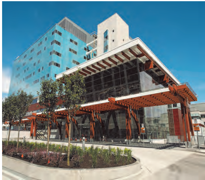
Critical Care Centre
