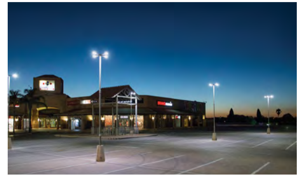
The cost-effective Skido LED luminaire illuminates the parking area at Atterbury Value Mart.
