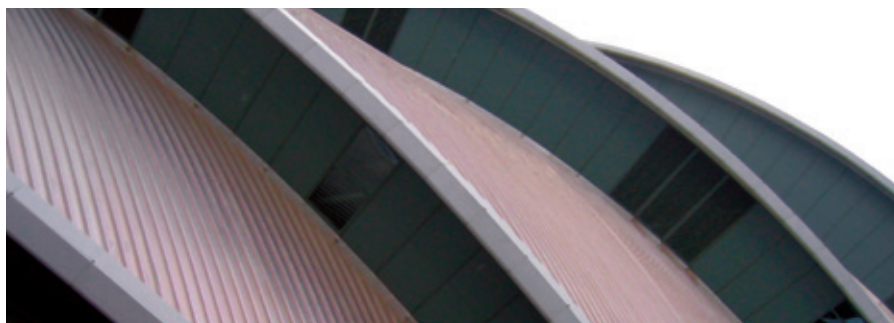
Titanium cladding at the Clyde auditorium, Scotland
