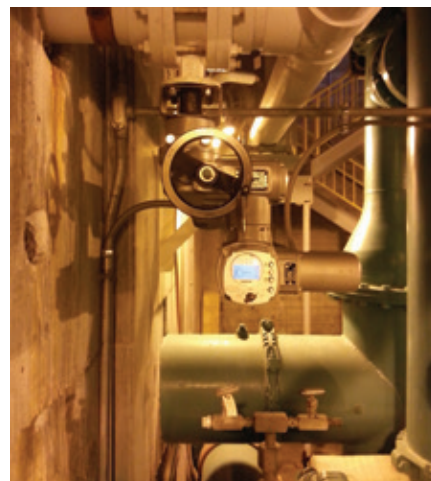
Auma intelligent actuators retrofitted at the Shoshone Municipal Water Treatment Plant
