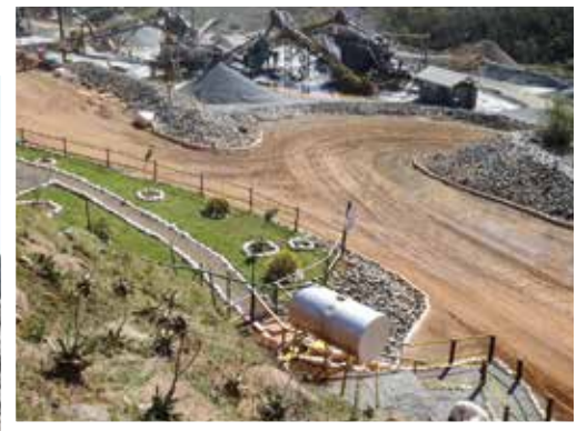
Midmar Crushers' pedestrian walkways and garden (Alan Cluett).
