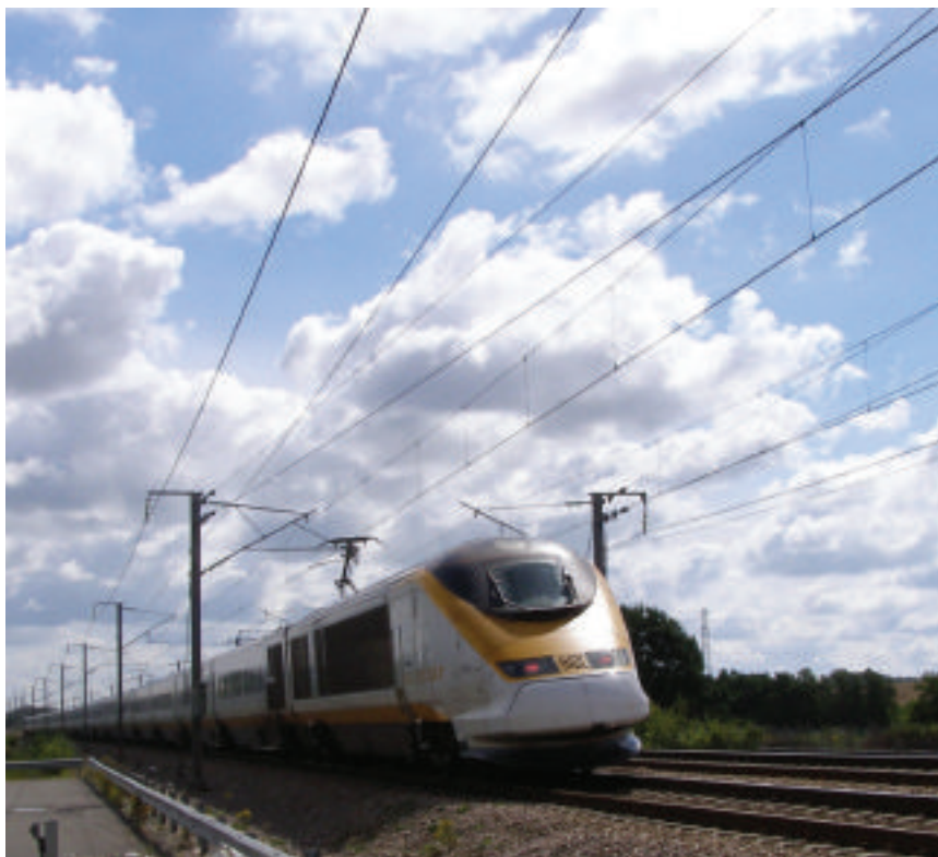
▲ Courtesy of a channel tunnel rail link upgrade incorporating RFS's ClearFill 'Line' solution, trains can now travel at 230km/h from England's coast right through to London
