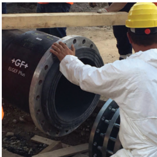
GF supplied eight ELGEF electrofusion couplings
