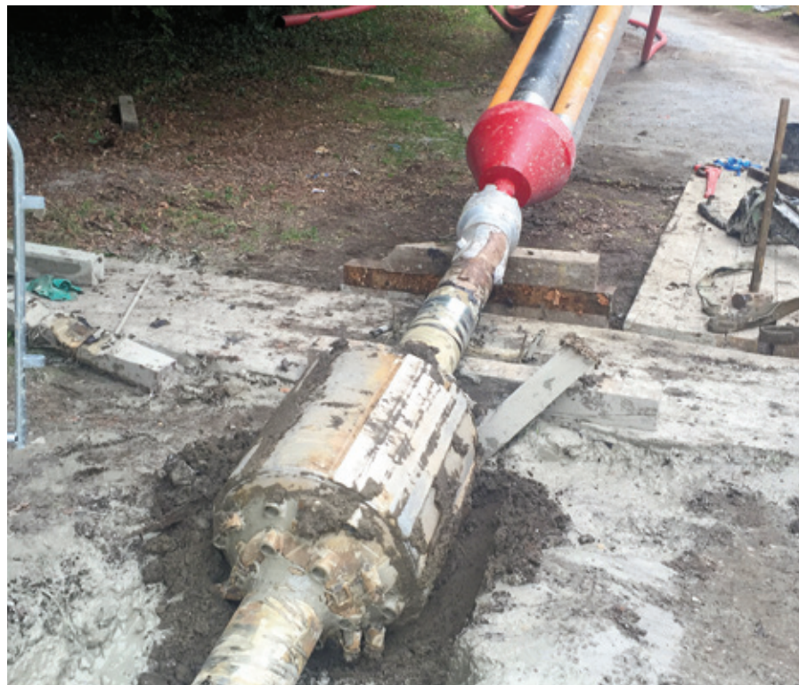
Detail of the final reamer/towing head/pipe bundle assembly
