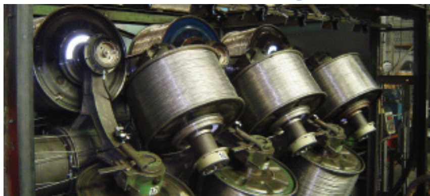
○ Typical placement of wire break detection monitors
