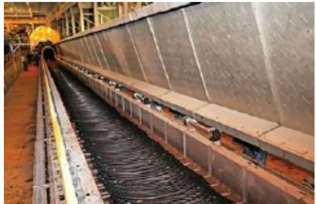
○ Emirates Steel is the largest integrated steel producer in the UAE
