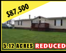
$87,500 MLS# 55040 - MAX MEADOWS - 3 bed 2 bath home on 5 acres already fenced for horses! Bonus room attached to master BR, FP, wood-burning stove, covered back porch with mountain views. 5.12 ACRES REDUCED
