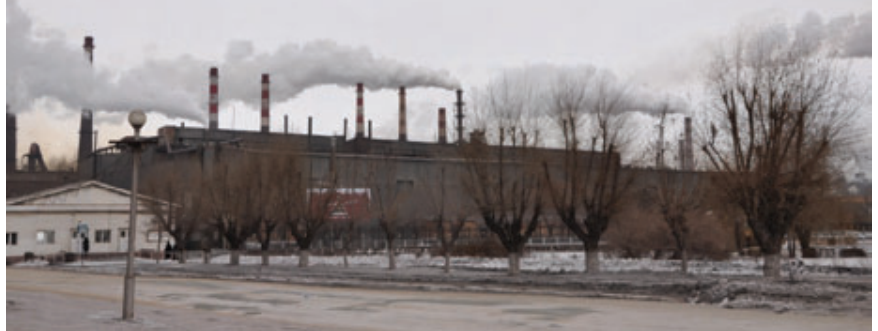
Imatek has installed a new factory to test steel pipe in Russia
