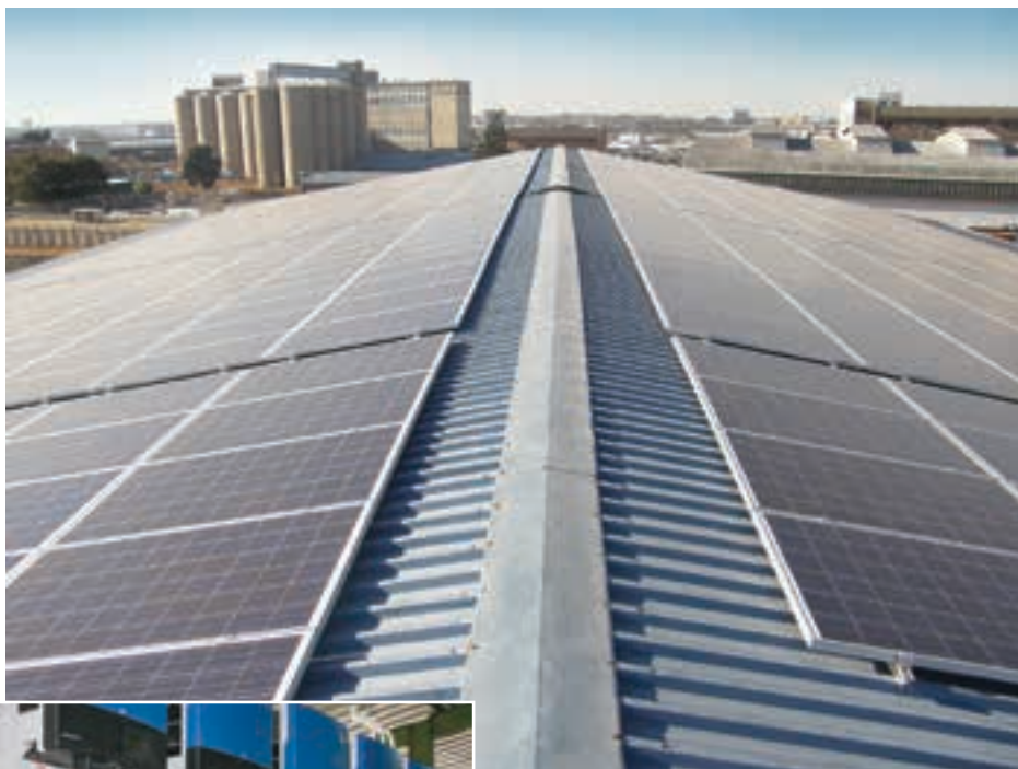
Above: The voestalpine Isando facility has 1 384 photovoltaic panels installed across the north-facing roof spaces. The panels provide a low-maintenance solution that will last 25 years.
