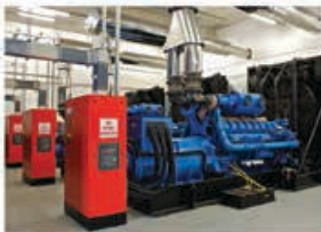
Six 2 000 kVA open type synchronising generator sets
