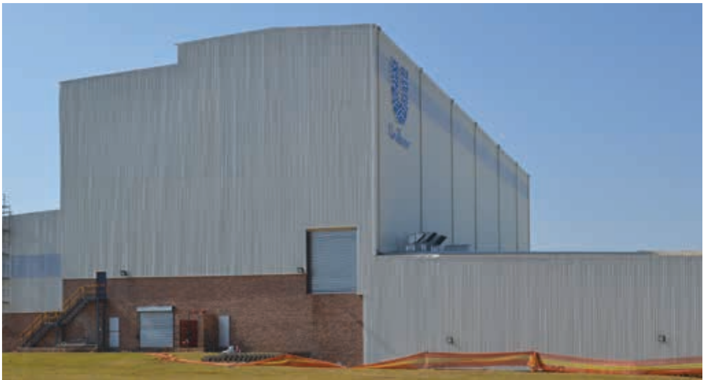
Unilever's new R1.4 billion Khanyisa Home Care factory in Boksburg.
