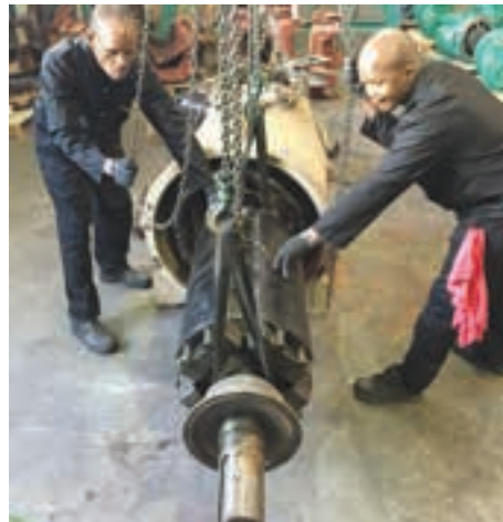
The removal of the rotor from a 1 650 kVA alternator with a failed stator at Vert Energy's Meadowdale premises in Edenvale, Gauteng. The unit is being stripped and checked to ensure there is no damage to the rotor.
