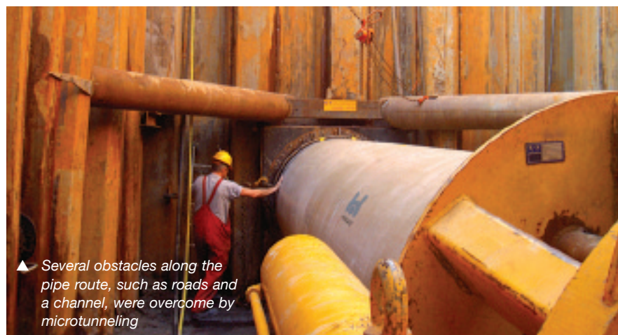
▲ The Hobas flush couplings used for jacking are leak tight and facilitate assembly
