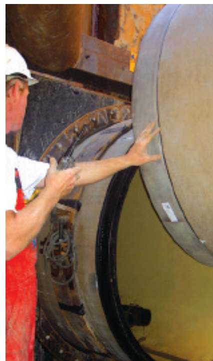
▲ The Hobas flush couplings used for jacking are leak tight and facilitate assembly
