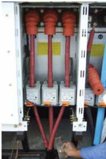
Figure 14: Illustration of the correct earthing for ring type CTs on each cable core used for overcurrent and earth fault detection.
