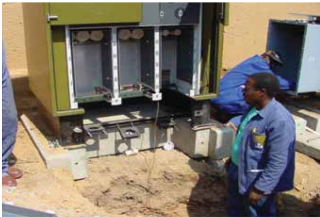
Figure 17: Example of SF6 RMU with an additional raising plinth and removable front sections.
