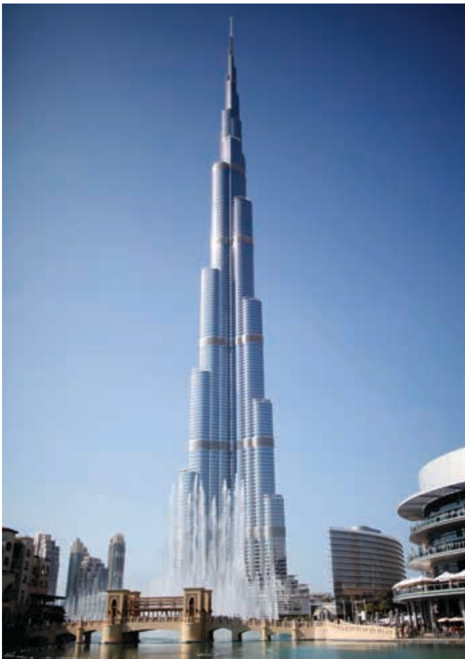
Burj Khalifa in Dubai, UAE, stands at 828 m tall, which results in a unique set of challenges for cable-based elevator systems, which generally offer a maximum ride height of up to 400 m.
