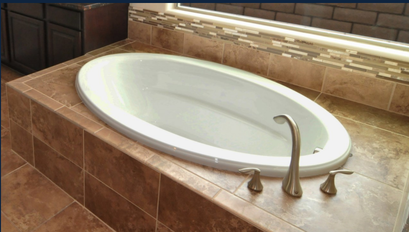
Soaking Tub with ceramic tile decking and skirting
