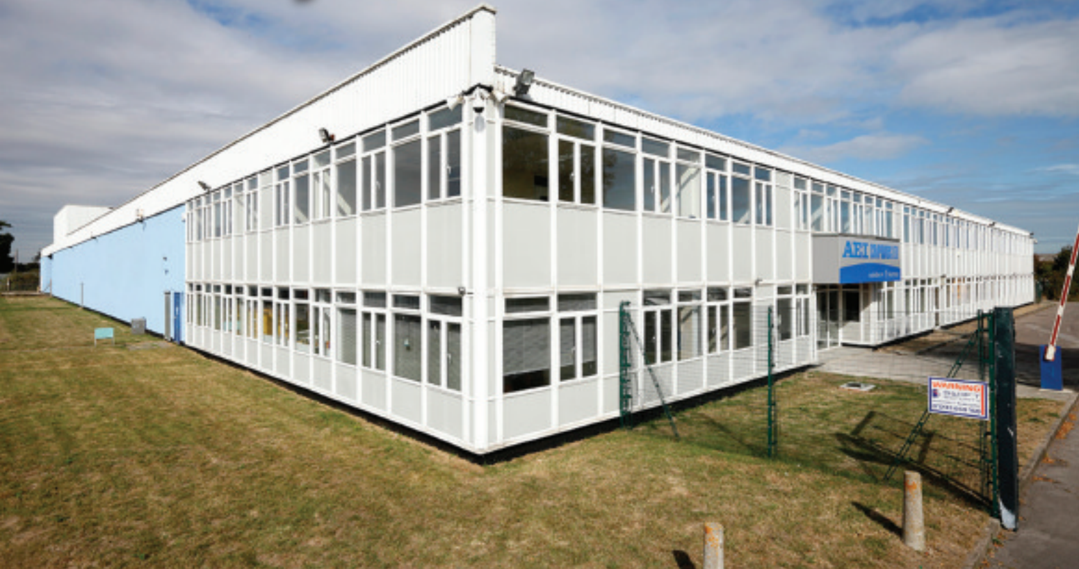
○ AEI Compounds facility in Kent, UK
