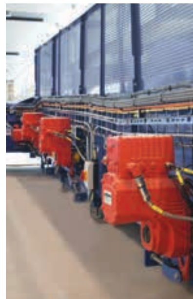
MoviGear combines a permanent-field synchronous motor, gear unit and electronics into a single housing, making it easy to integrate into a conveyor drive system.
