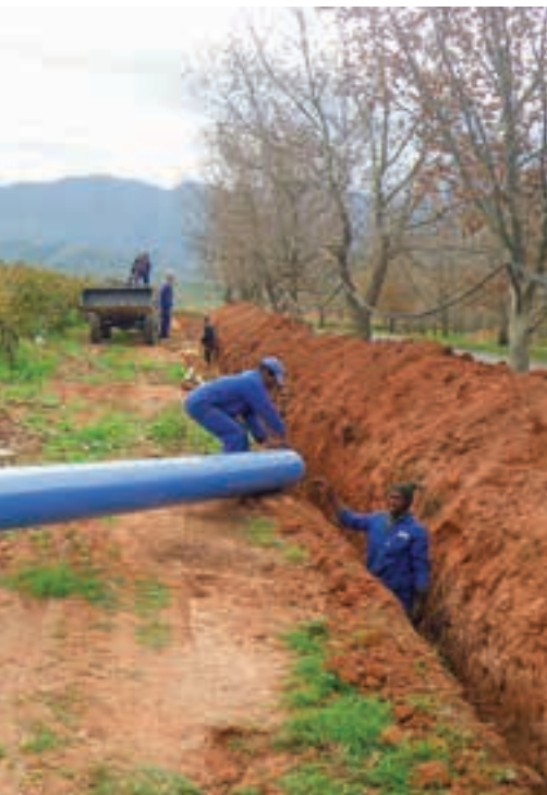
Above: Pipelines can sometimes be several kilometres long, it is therefore beneficial to test the pipeline in sections.
