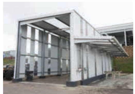
The MAN assembly plant has also installed a wash bay with a water recycling system, which includes an oil-water separator. The system captures rainwater from the roof for use to clean vehicles and to test truck cabs off the assembly line for leaks.
