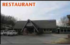
Established restaurant w/ stream on golf course in Roaring Gap, NC. Main level 6000 SF w/ kitchen, 2 DR, bar, dance floor, office, waitress stations, small cafe, outdoor patio. 2nd level 2100 SF catering kitchen, private DR. $440,000
