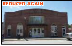
Updated building 9,359 SF on E Main St. Downtown Elkin. Part of building occupied by the Elkin Tribune, majority of lower level is vacant. $34,73 SF $200,000
