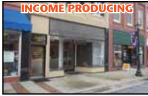
Income producing, restored, HW floors, 13'9" ceilings on W. Main St. downtown Elkin. Main level 2,840+/- SF. 2nd level has 2 furnished residential lofts. $299,000
