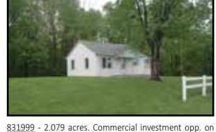
831999 - 2.079 acres. Commercial investment opp. on main thoroughfare in Elkin across from Super Wal-mart, Zaxby's and shopping mall. House being sold "as is where is." Possibility of leasing dwelling as interim use. $135,000
