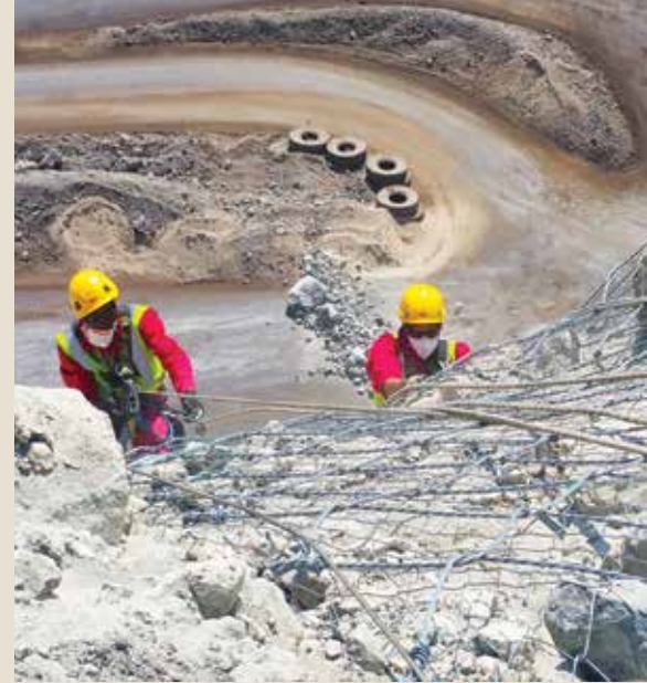
Installation of the QUAROX® PLUS rolled cable net.
