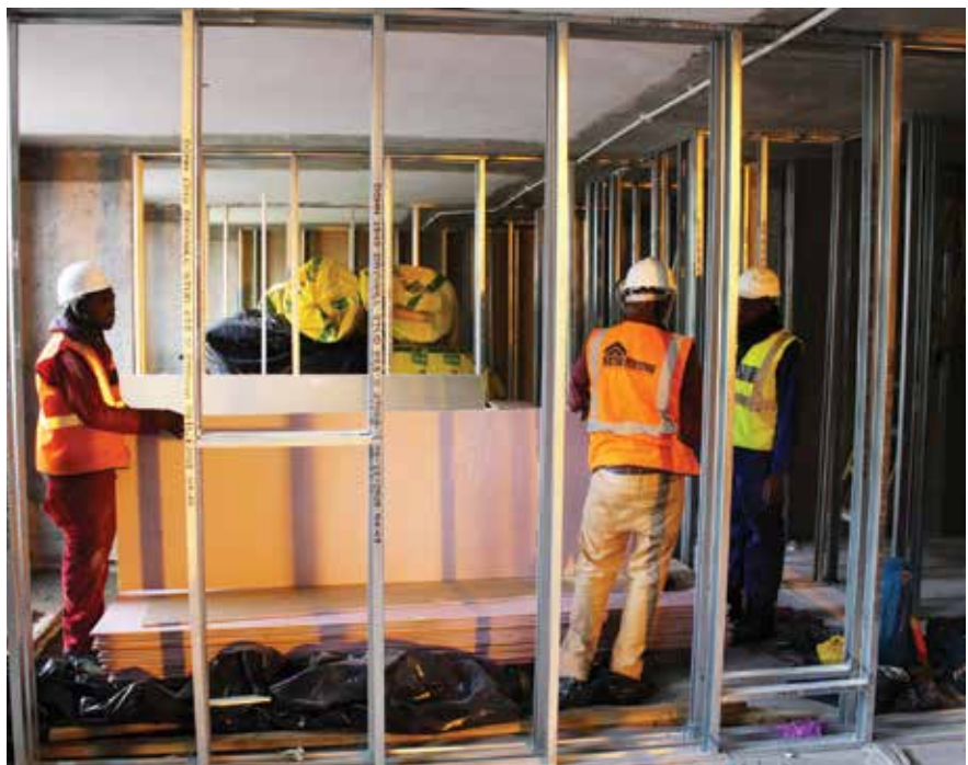
Subcontractors start with the installation of the services components of the structure and then install the dry-walling, ceilings, doors, tiling and skirting.
