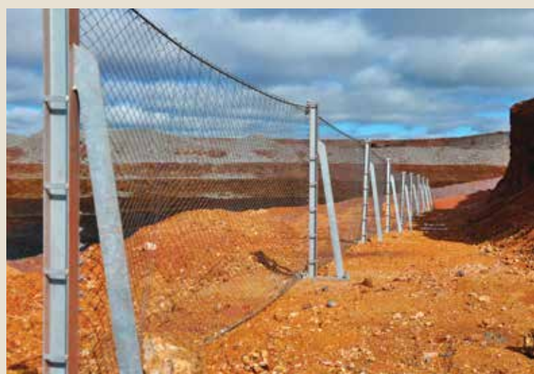
GBE barrier during installation showing mesh panels pre-installed at factory.
