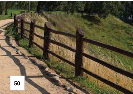
H3 – Moderate Hazard: Outside above ground, subject to periodic wetting and leaching (cladding, decking, stairs, balustrades, log homes, etc.)
