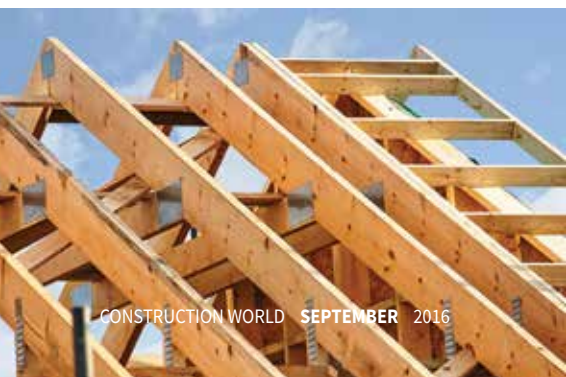
H2 – Low Hazard: Inside above ground, protected from wetting and leaching (roof trusses, framing, panelling, laminated beams, flooring, etc.)
