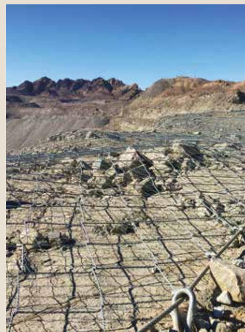
QUAROX® PLUS draping system is a cost-effective mitigation solution.
