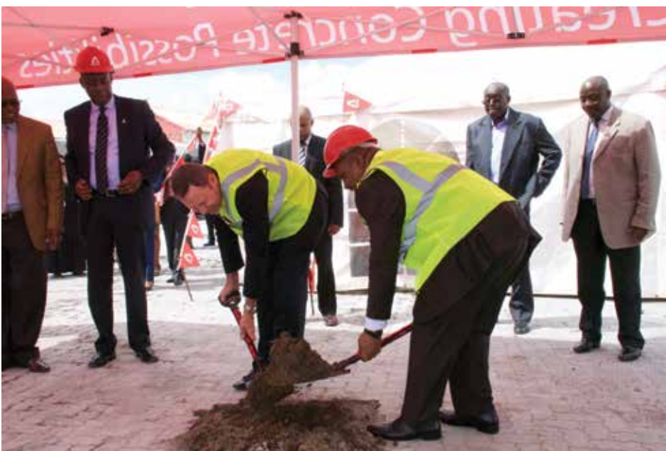
Minister of Trade and Industry of Lesotho, Honourable Joshua Setipa (far left) with AfriSam CEO, Stephan Olivier (centre) and the Deputy Prime Minister of Lesotho, Honourable Mothetjoa Metsing (right), officiating at the ground-breaking ceremony.
