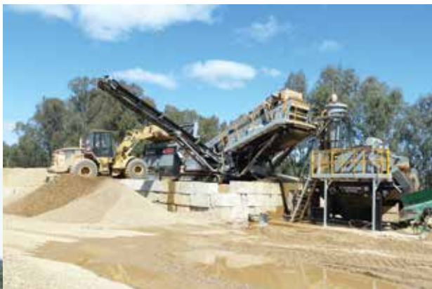
Mawsons' Cat 950G wheel loader feeds the M1700 rinsing screen (centre), which in turn feeds the FM120C compact cyclone wash plant (right).
