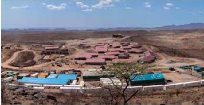
Site of the Lake Turkana Wind Farm. Photograph courtesy of Lake Turkana Wind Farm
