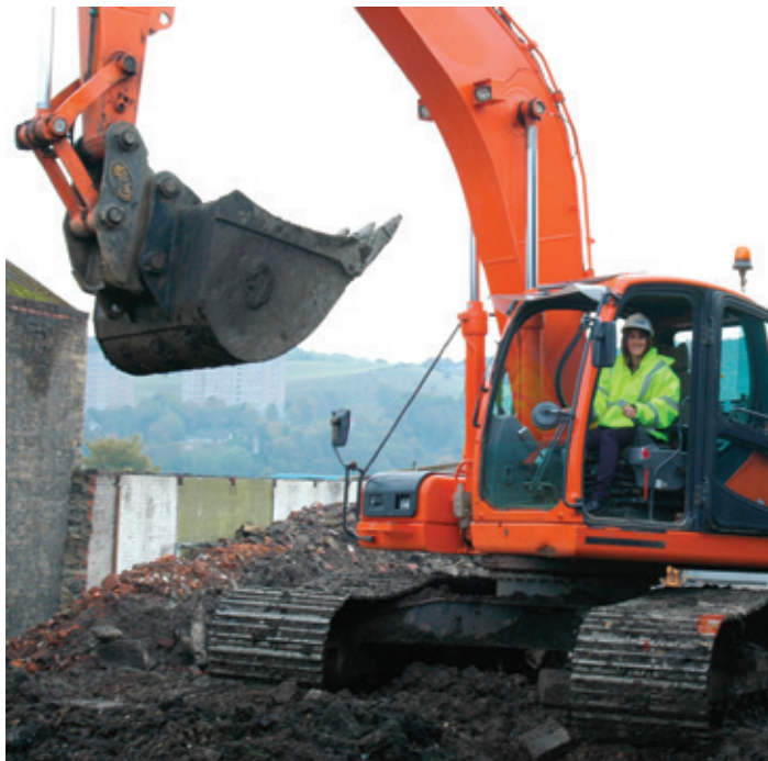
▲ Managing director Debbie Mellor takes control during the construction
