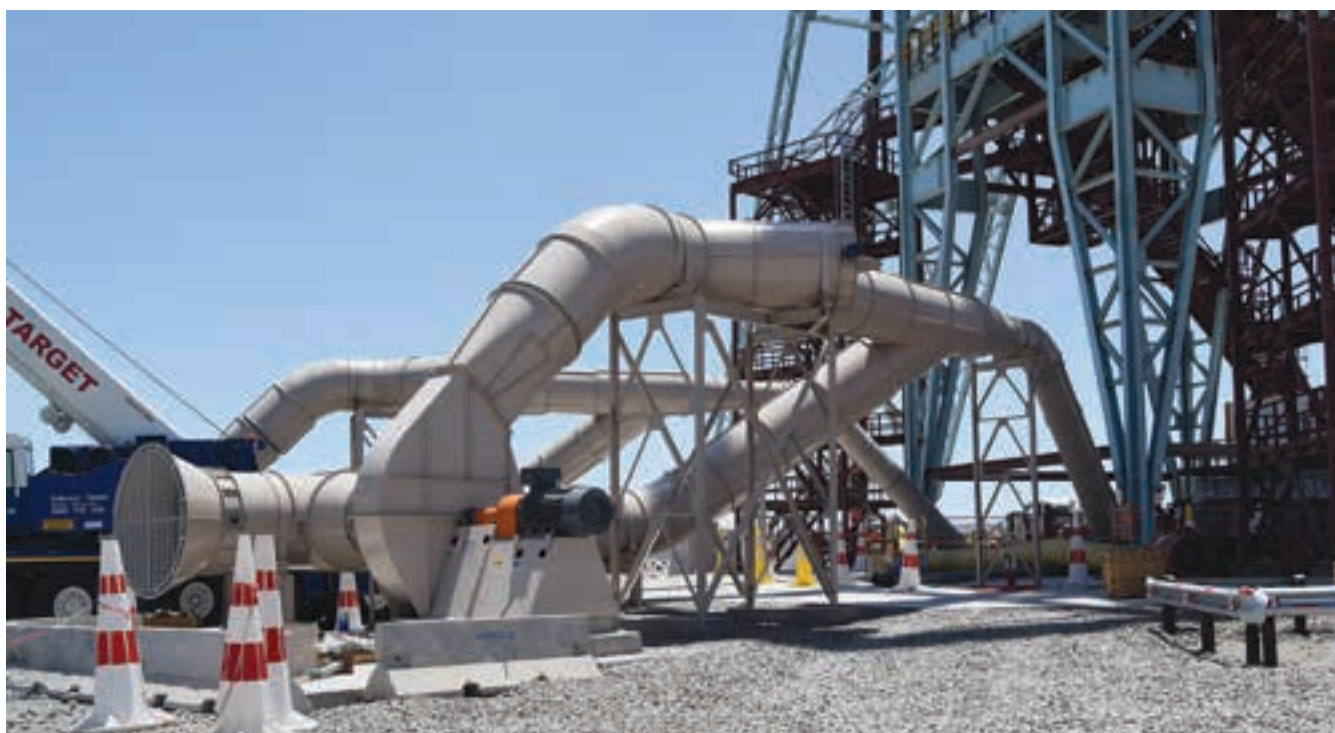
Ventilation system for the service shaft.
