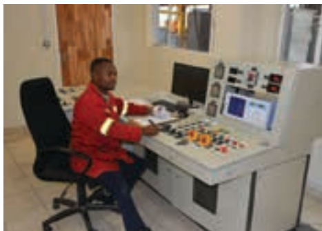
100 MVA 132 kV Testing Bay
