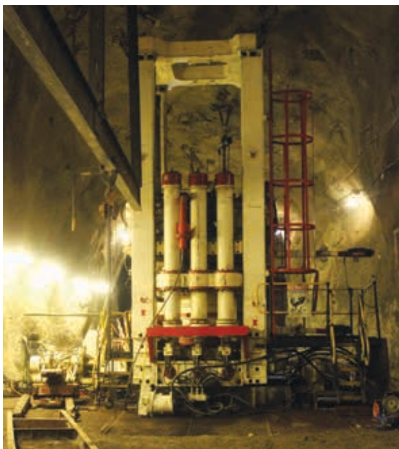
A Murray & Roberts Cementation raise borer working underground at Palabora.
