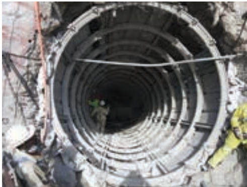
Becker Mining South Africa's steel arch support systems are designed for use in friable ground in tunnel applications, including haulages, incline shaft portals and special shafts.
