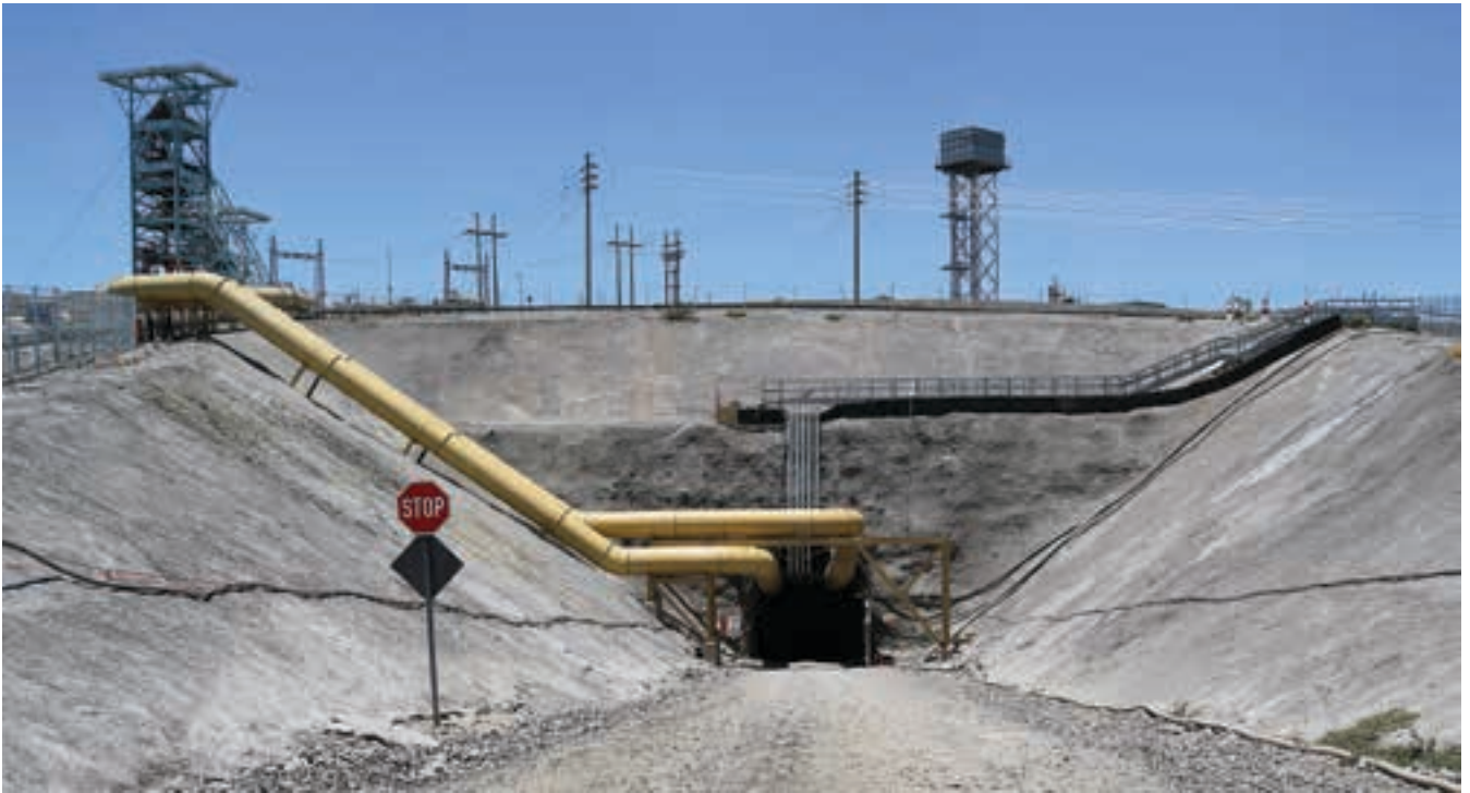
The portal of the decline. Ultimately the decline will have a length of 7 km.
