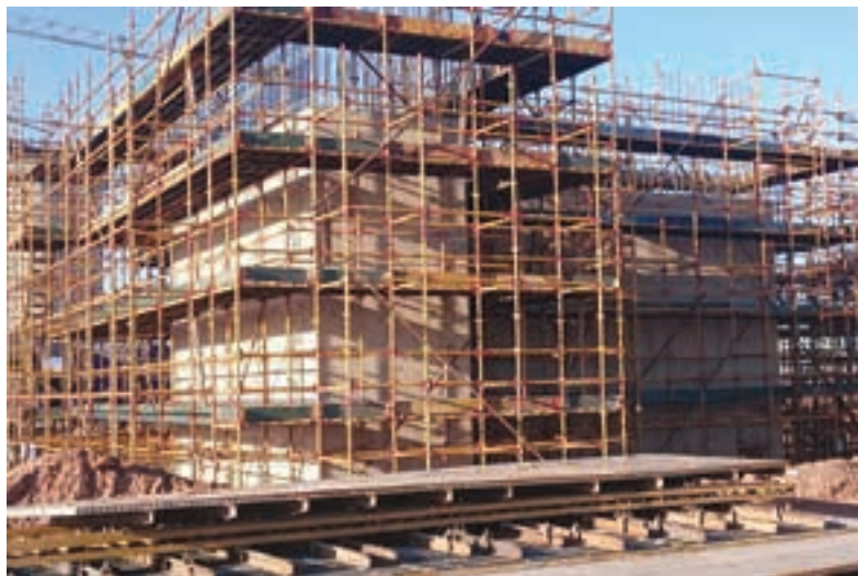
The bases for the mills under construction.
