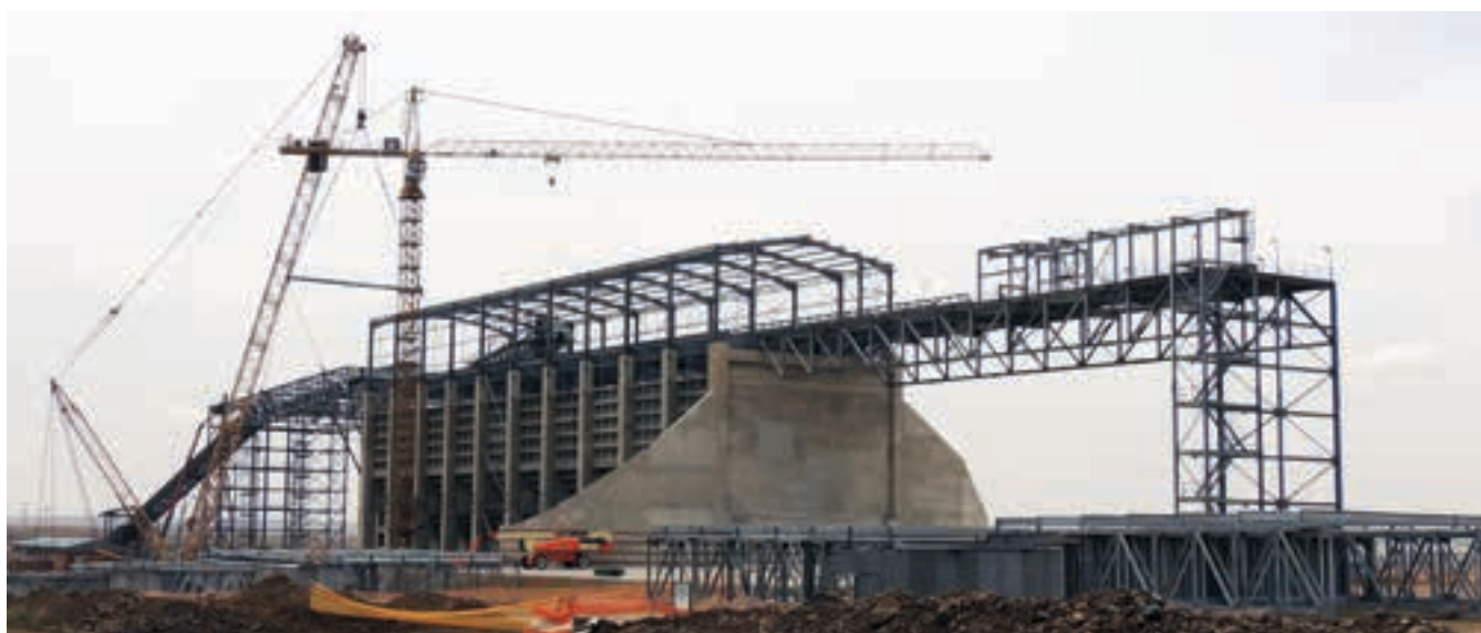
Shondoni’s 15 000-ton capacity surface coal bunker under construction; the design included both precast and in-situ concrete elements.
