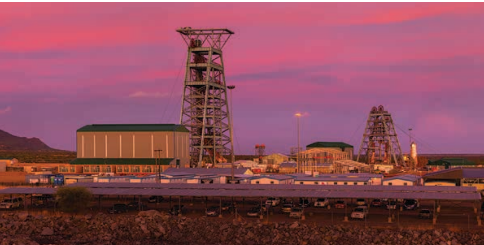
Wesizwe's Bakubung Platinum Mine (BPM), one of WorleyParsons' current South African projects.
