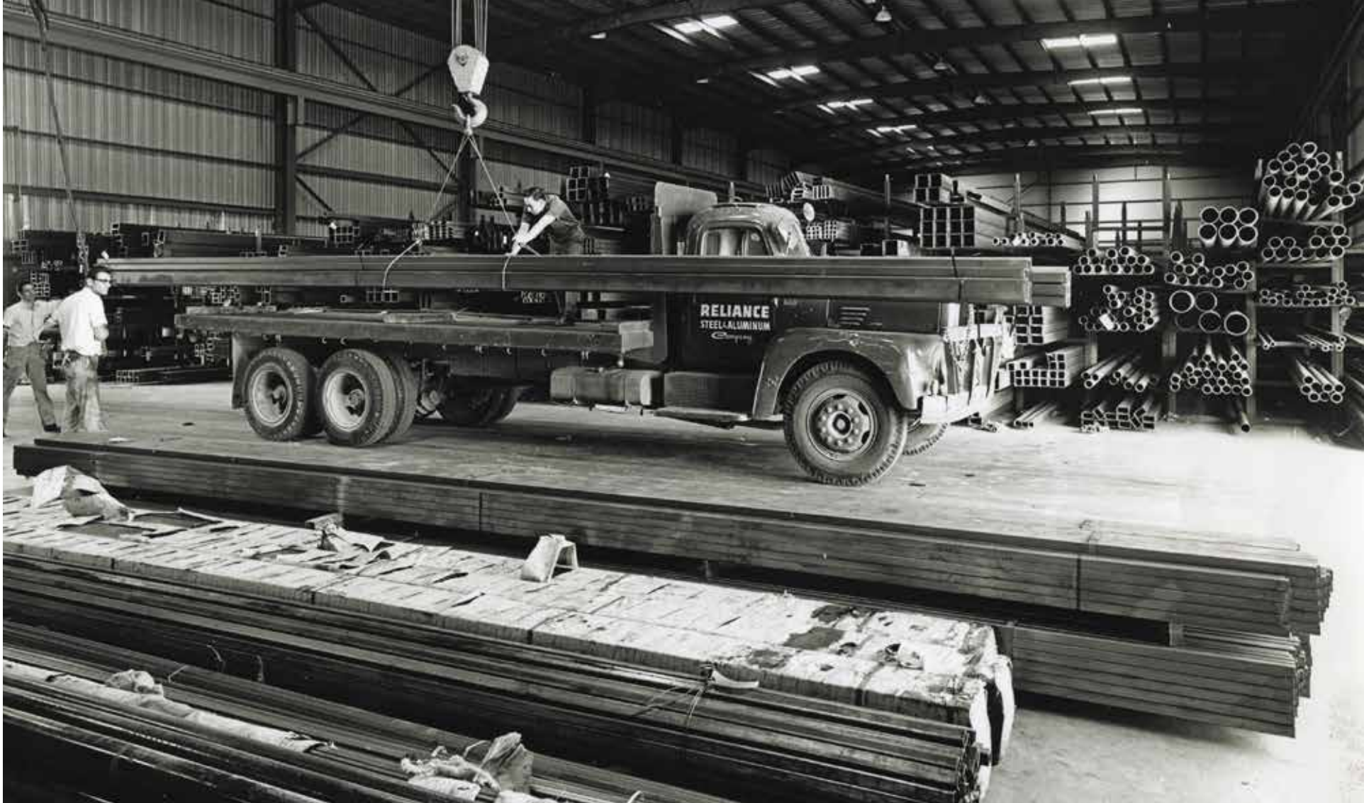
Loading up square tube steel for delivery around 1960.
