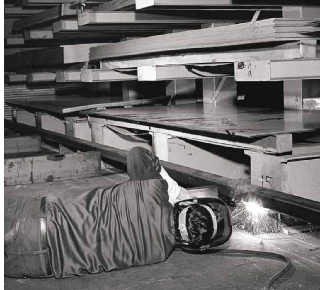
As soon as Reliance acquired new facilities, arrangements were made for improved storage and handling. Here an employee installs rails for a "sideloader" truck at the Santa Clara service center.
