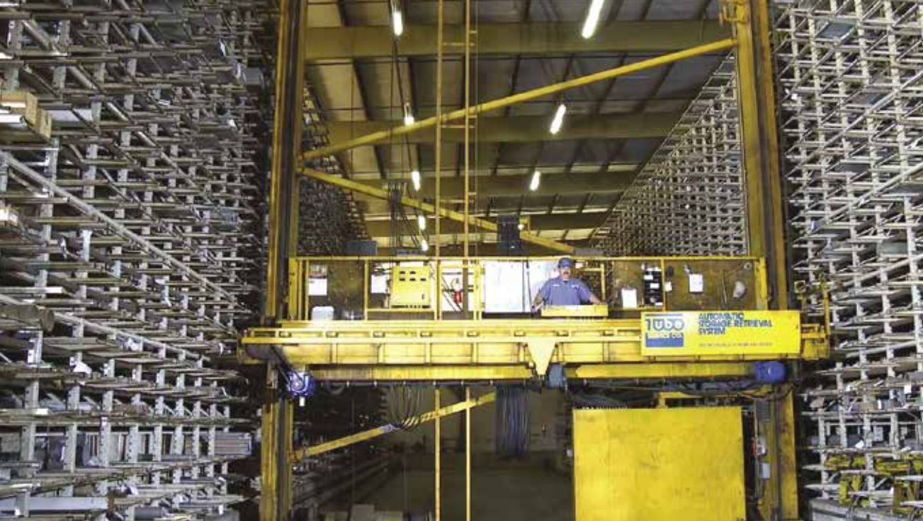
Bill Gimbel's early 1960s invention had come a long way by 1988, when Reliance division Tube Service Co. installed the first automatic storage and retrieval system of its kind.
