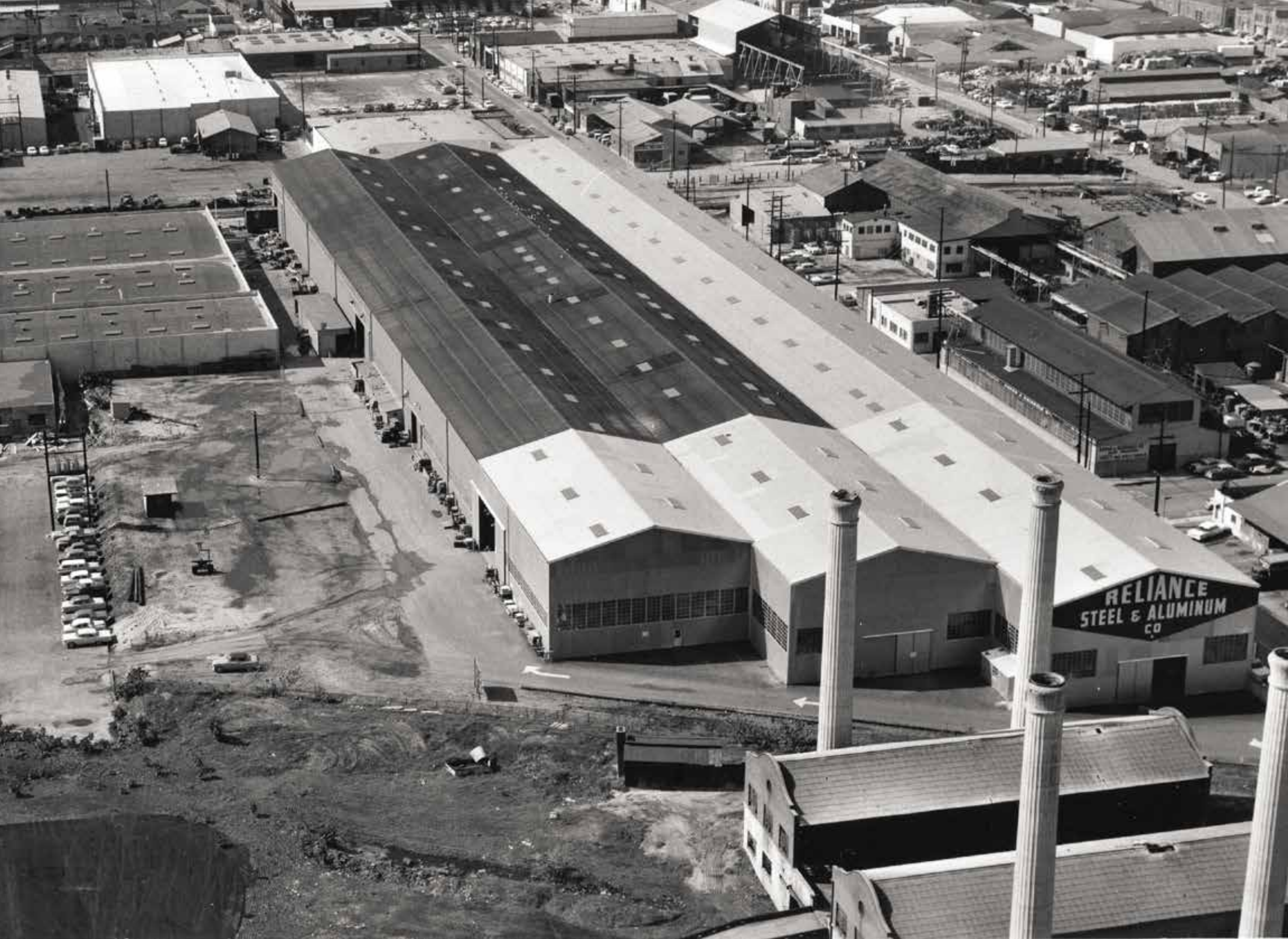
An aerial view of Reliance's now-expansive flagship facility, featuring three bays and an office building, on 26 th Street in Vernon, California, about 1960.
