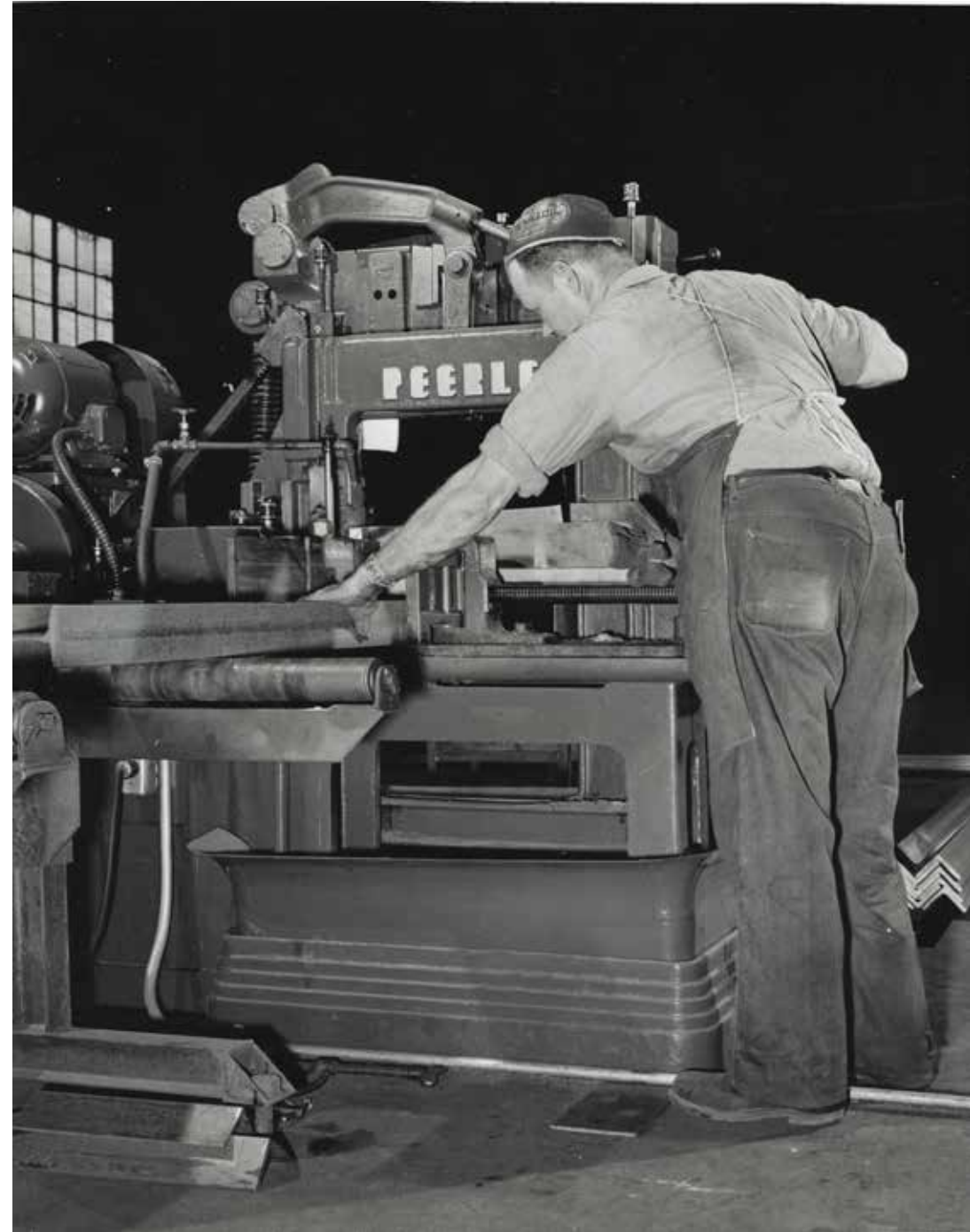
Preparing to cut an I-beam with a Peerless heavy-duty power hacksaw.
