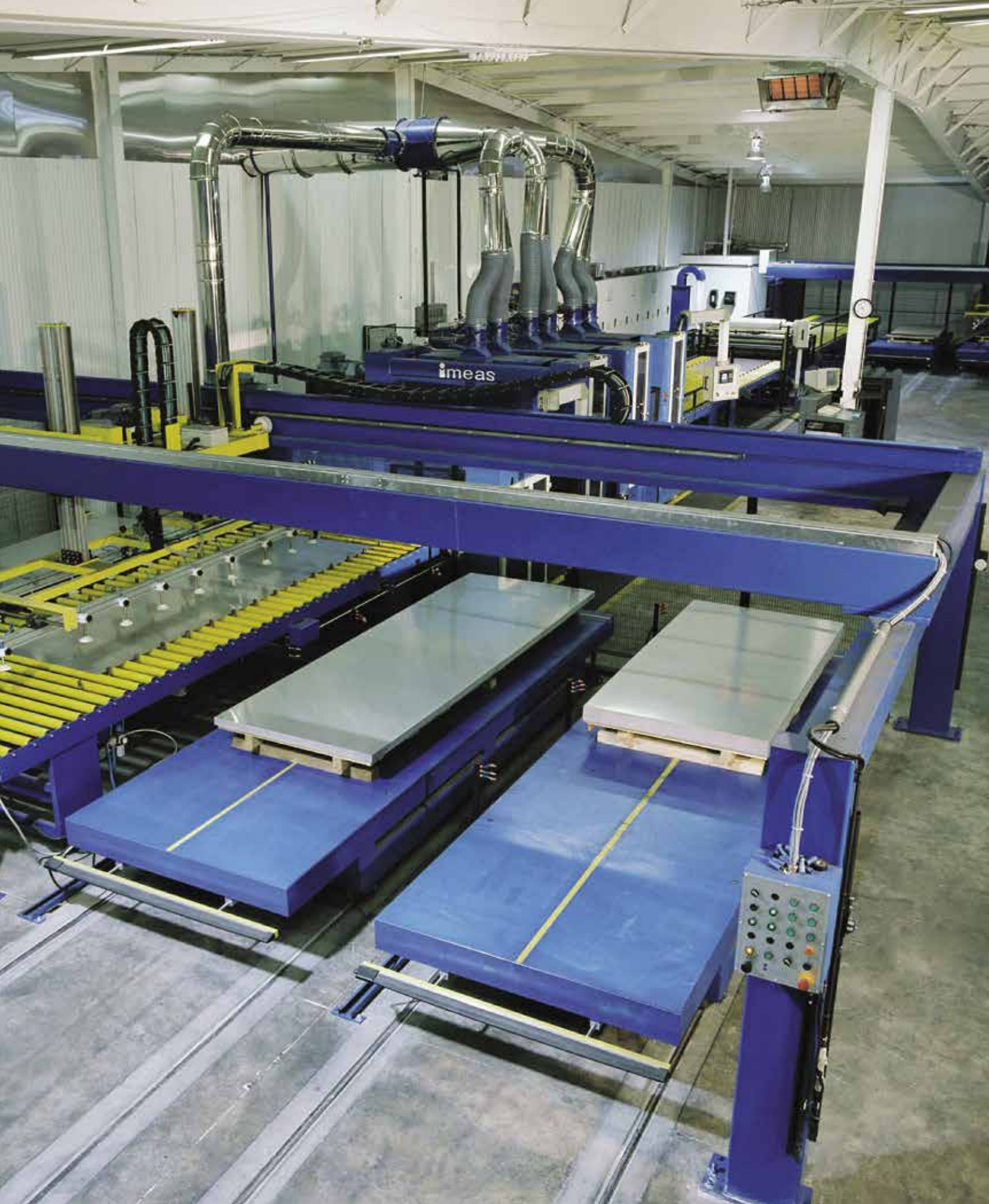
The sixty-inch, fully automated polishing line at the Atlanta, Georgia, warehouse of Phoenix Metals.
