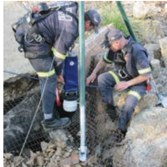
The shaft camera being lowered down an abandoned mine to check the water level in the shaft.
