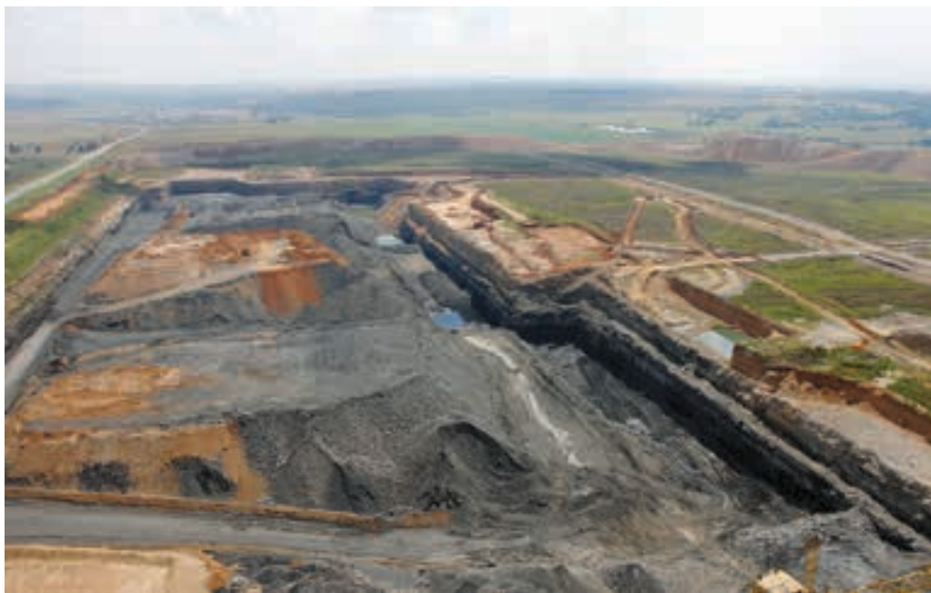
An early shot of opencast mining operations at Zibulo, which was officially opened in 2012.
