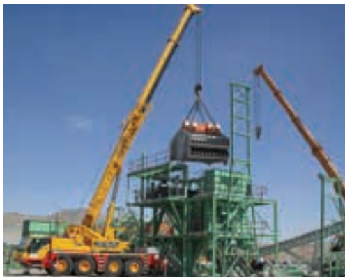
A Joest vibrating screen being installed for a gold application in Namibia.
