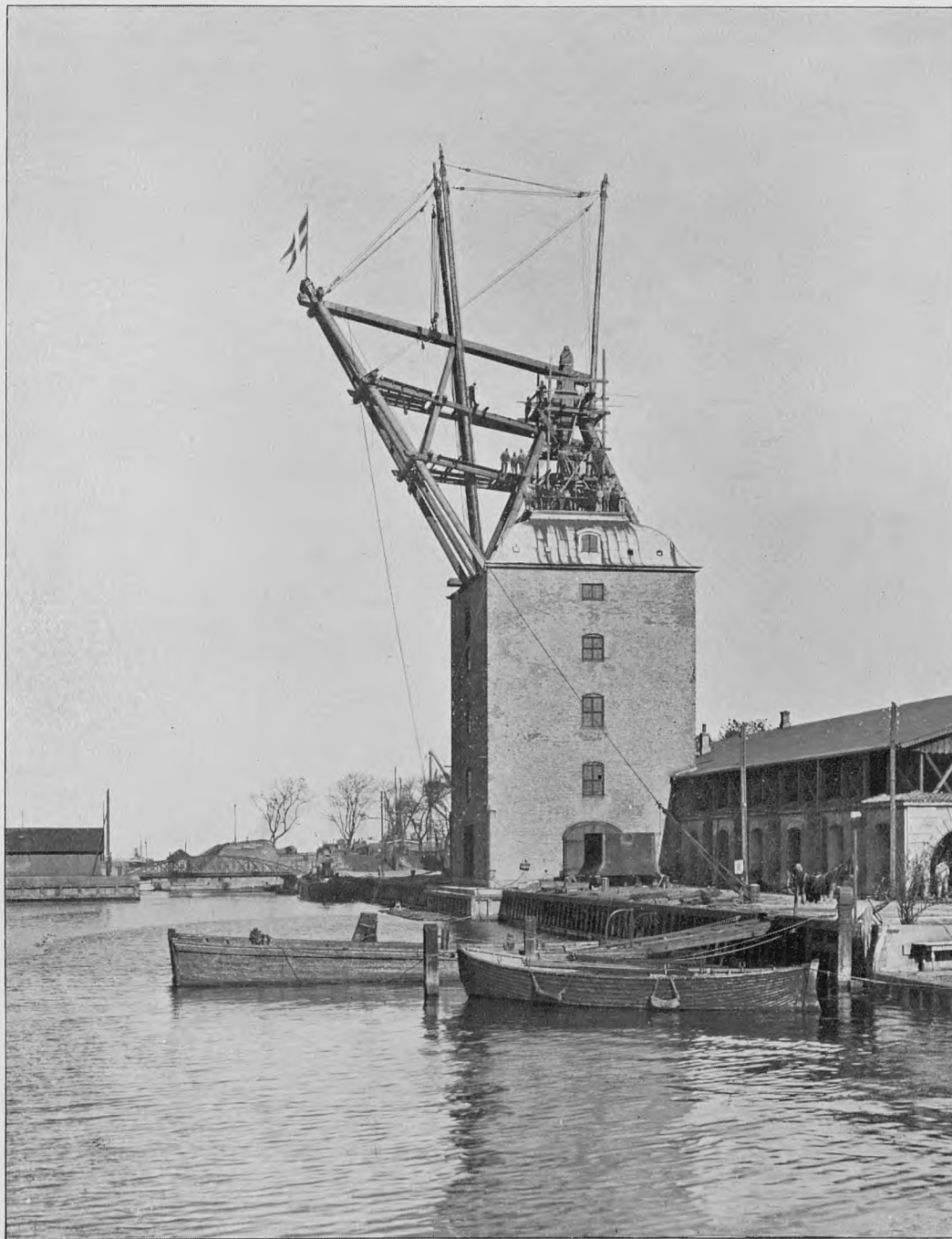
Nyholms Krans Hovedreparation, 1922.
