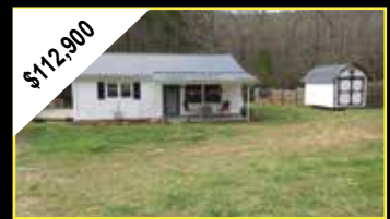
$112,900 MLS# 63492 FORT CHISWELL 2BD/1BA home with metal roof, updated bath, eat in kitchen, large living, and large deck and porch. Creek out back spanning back side of property, outbuilding, privacy fencing.
