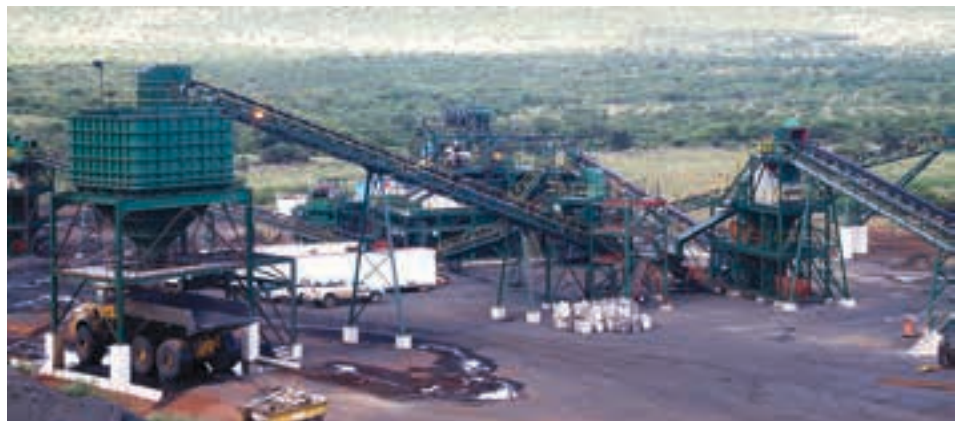
The new coal processing plant has a 50-ton per hour capacity.
