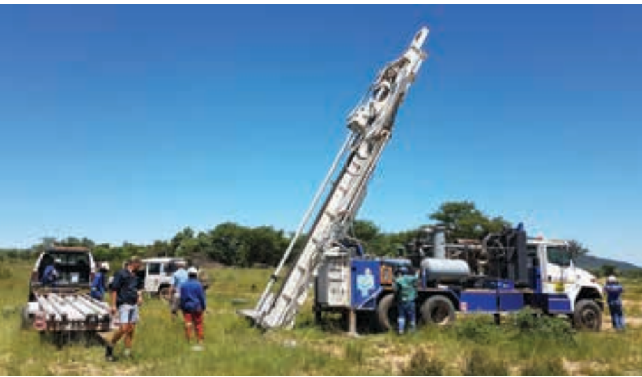
Preparing for percussion drilling at Frischgewaagt.
