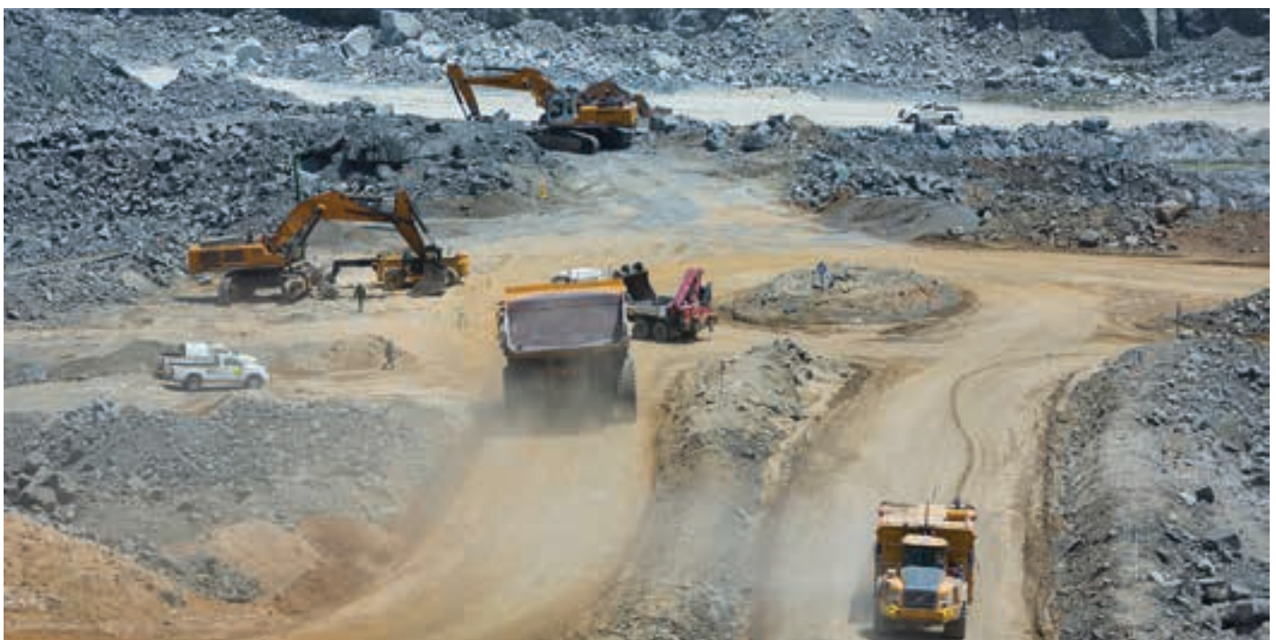
Open-pit operations at the Tharisa mine (photo: Tharisa Minerals).
