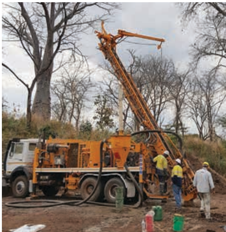
Drilling at Lindi Jumbo in 2016 (photo: Walkabout Resources).
