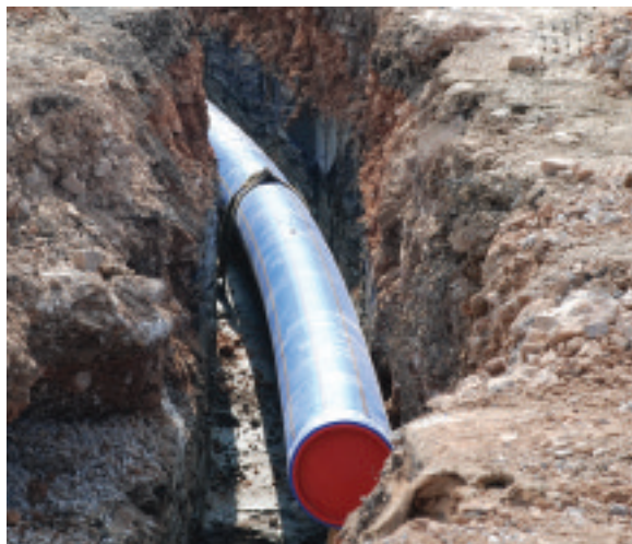
▲ Protecta-Line incorporates an impermeable aluminium barrier layer within the polyethylene
