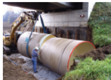
▲ The first phase, from the intake works Penz in Aichdorf to the Pöls Bridge
