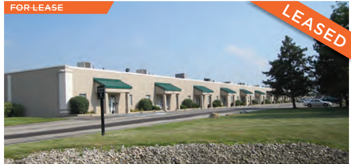
Lincoln Business Park 10,800 sf 1327-1441 Sadlier Circle West Drive, Indianapolis, IN
