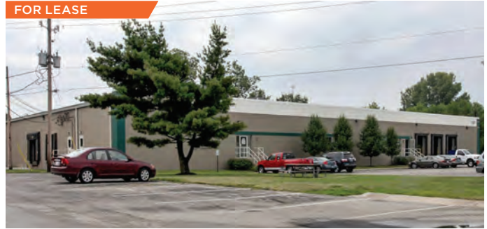
Lincoln Business Park 15,000 sf 1367 Sadlier Circle South Drive, Indianapolis, IN
