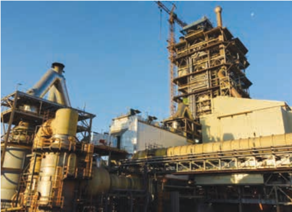
The new Kansanshi smelter is expected to process 1,2 Mt/a of concentrate to produce over 300 000 t of copper metal once in full operation (photo: FQM).
