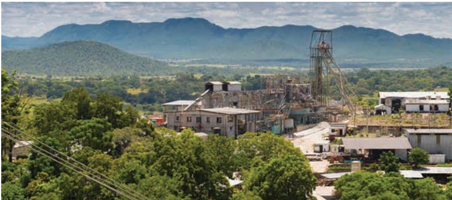
Metallon's Shamva mine, where underground mining first started in the 1890s. It is Metallon's second biggest producer after How mine (photo: Metallon).
