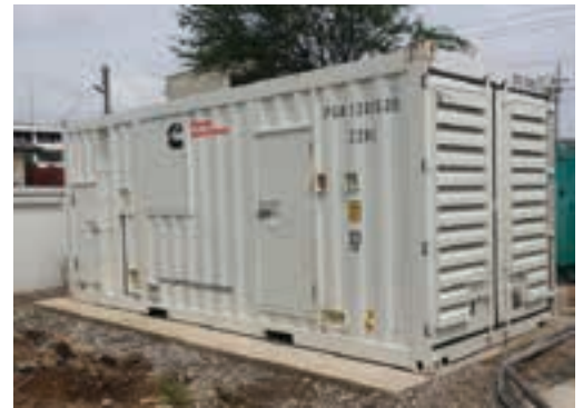
One of the containerised Cummins C700 D5 units for the Ghana District Hospital Programme. Below: the 700 kVA standby units offer greater fuel efficiency and lower maintenance costs.
