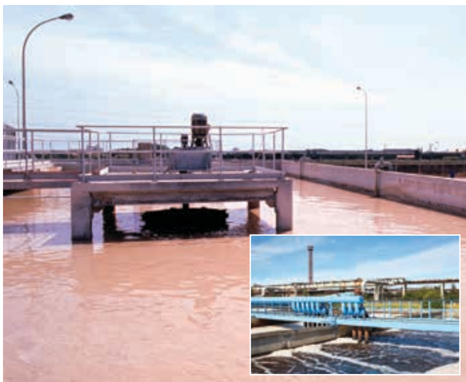
Wastewater aeration using oxygen versus air significantly lowers VOC emissions by reducing gas stripping. Air Products' Oxy-Dep range of technologies provide efficient oxygenation (usually >90% oxygen transfer efficiency), where high loads exist. Oxy-Dep also provides a reduction in odours, surface foaming, aerosols and VOCs, as well as improved sludge settling and dewatering, either when retrofitted or in a purpose-built activated sludge plant. Inset: Traditional aeration (using air) associated with significantly more surface foaming.
