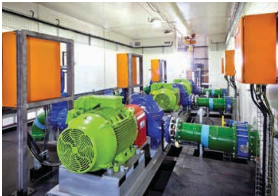
Four KSB Omega 200-420 A pumps were specified for Sishen’s modular pump station, each with a nominal flow capacity of 600 m 3 /h, giving a total flow capacity of some 2 400 m 3 /h into the 40 m head.
