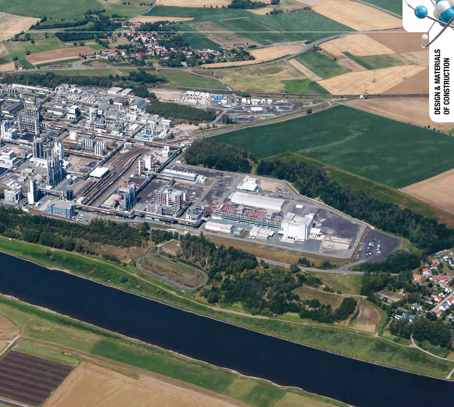
The Wacker Chemie Nünchritz site outside Dresden
