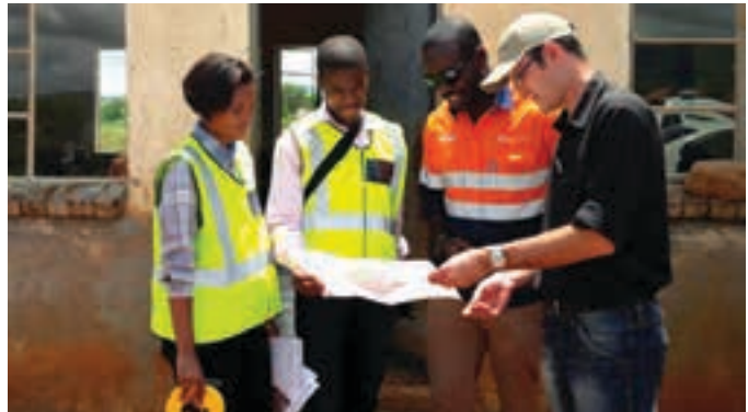
Seen on site during the Lesedi refurbishment project are (from left) Palesa Mabelane, graduate quantity surveyor; Luthando Jele, graduate quantity surveyor; Raphael Baiden, associate director mining and metals for Turner & Townsend; and Werner Botha, senior projects manager, Ivanplats.
