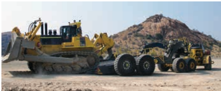
Loading a dozer onto a DB120 takes just minutes.
