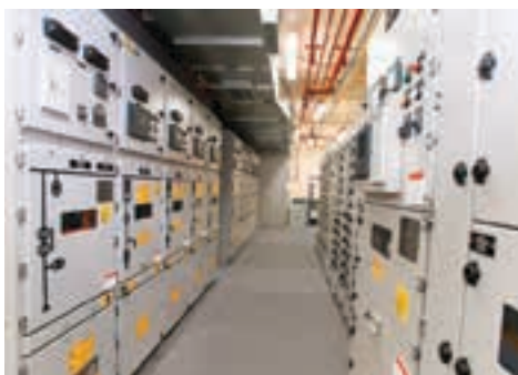
LV and MV Switchboards inside E-House
