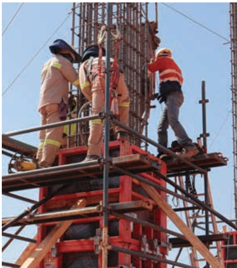
The concrete team pours the next section of the conveyor columns.
