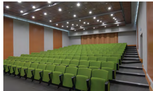
The BEKAQUAD and BEKA CUBO downlights ensure an even lighting level in the conference facilities.
